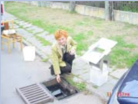
Malgorzata Witczewska, Deputy Director of Environmental Services, the City of Plock, inspects the installation of GreenTechTexas' EcoDrain storm water filtration system.
