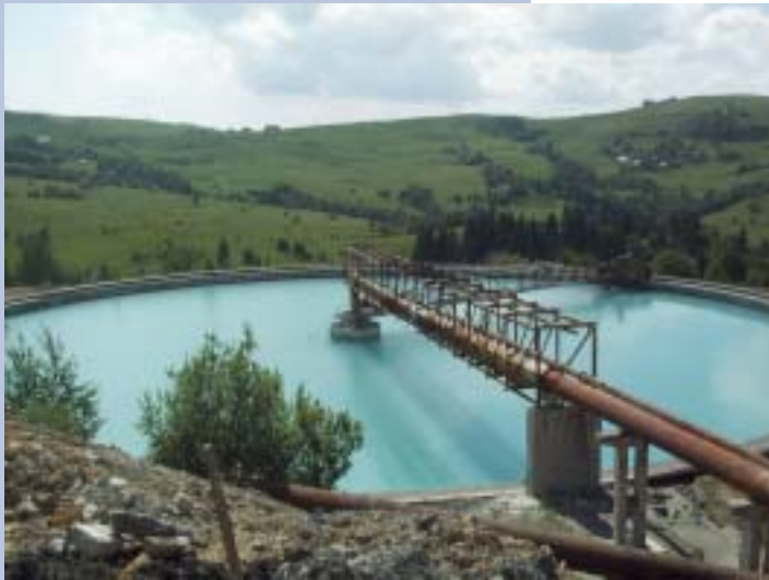
Mining sites throughout the region, like the one pictured above in Deva, Romania, are investing in cleaner production processes.
